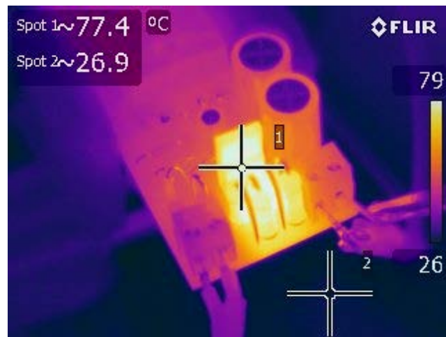
Figure 41 – 90 V VAC, 30 V LED Load, 0 V Dim. Spot 1: Pre-Load Switch (Q6): 77.4 °C.
