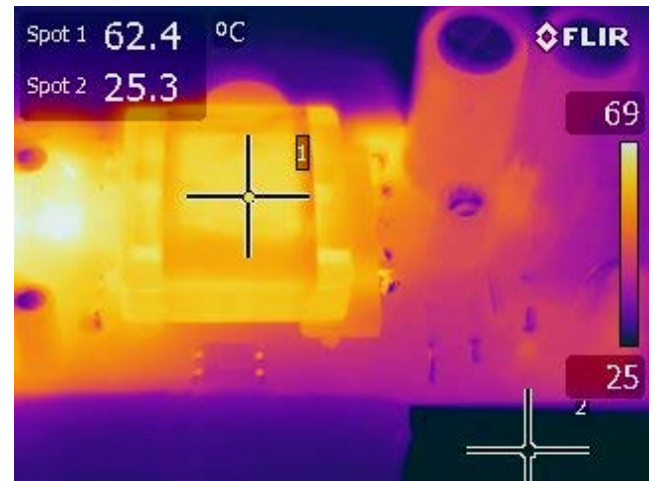
Figure 36 – 90 V VAC, Full Load. Spot 1: Transformer (T1): 62.4 °C.
